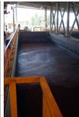
(Top) construction work proceeds on BWT DAF cells; (left center) DAF cell processing influent; (right) empty DAF cell—images taken Spring 2009 at Valdez Marine Terminal by Mark Morones, JPO/SPCO Information Officer
